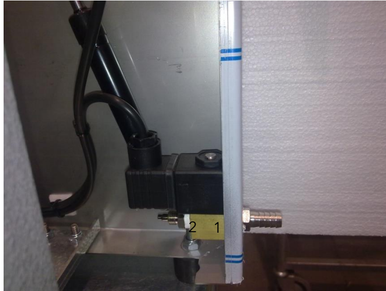
Figure 52. Solenoid valve inert gas injection models TVA410-430-432B2
